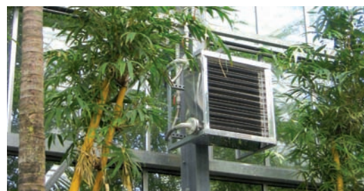
■ Water to air heating unit
