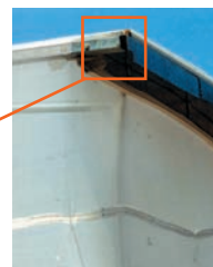
■ Insect-netting on multispan greenhouse roof vent
